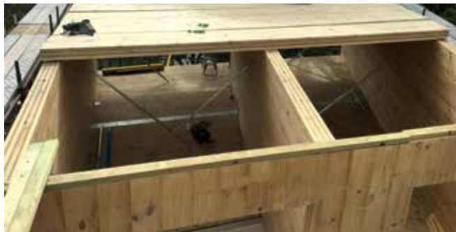
2D cross-laminated timber (CLT) panels: Xlam 12
